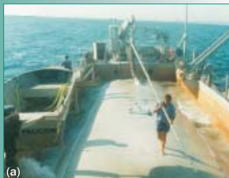
Figures 5.7 Filling (a) and placing (b) geotextile containers during construction of the Narrowneck multi-functional artificial reef, Australia (courtesy International Coastal Management)
