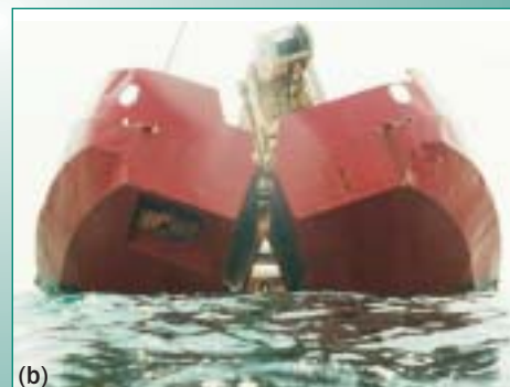
Figures 5.7 Filling (a) and placing (b) geotextile containers during construction of the Narrowneck multi-functional artificial reef, Australia (courtesy International Coastal Management)
