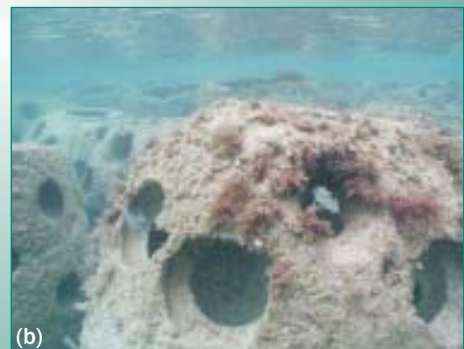
Figures 5.5 (a) and (b) Submerged breakwater comprising Reef Ball™ units in Grand Cayman (courtesy L Harris, Florida Institute of Technology)
