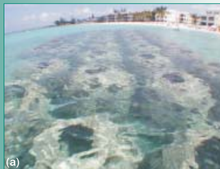
Figures 5.5 (a) and (b) Submerged breakwater comprising Reef Ball™ units in Grand Cayman (courtesy L Harris, Florida Institute of Technology)
